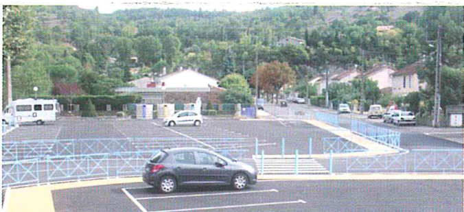
Le parking place Kennedy, flambant neuf.
